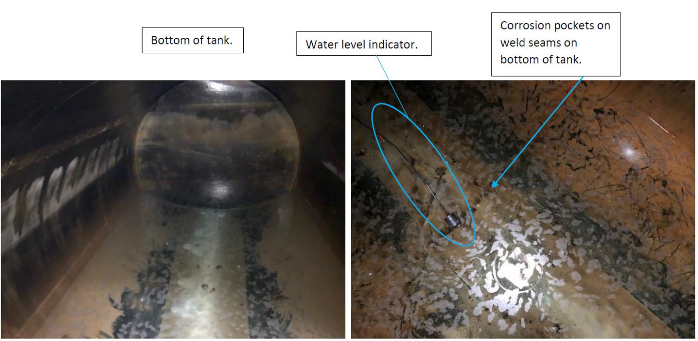
Interior of Tank – October 2018
