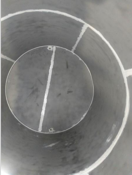
Interior of Tank – Post Sandblasting
